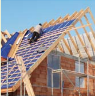
Heat pumps in new buildings. Independent of oil and gas
