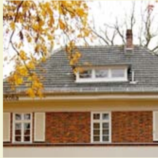
Heat pumps for modernisation of existing buildings. Combination with existing heating appliances
